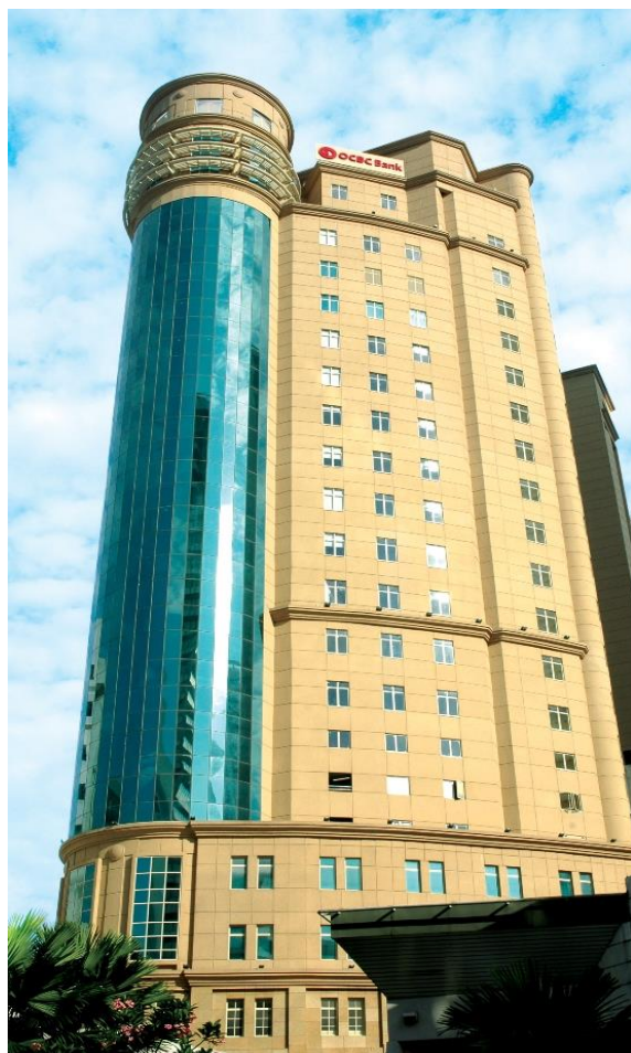
Menara OCBC, headquarters of OCBC Bank (Malaysia) Berhad.
