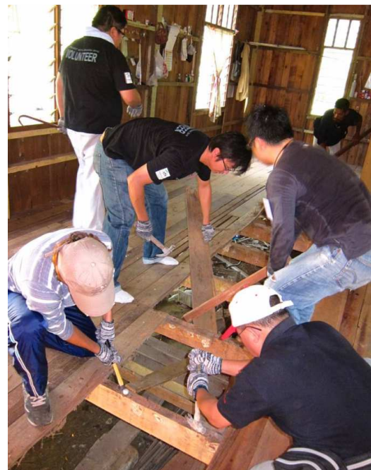
OCBC Bank employees replacing the floor boards of the house.
